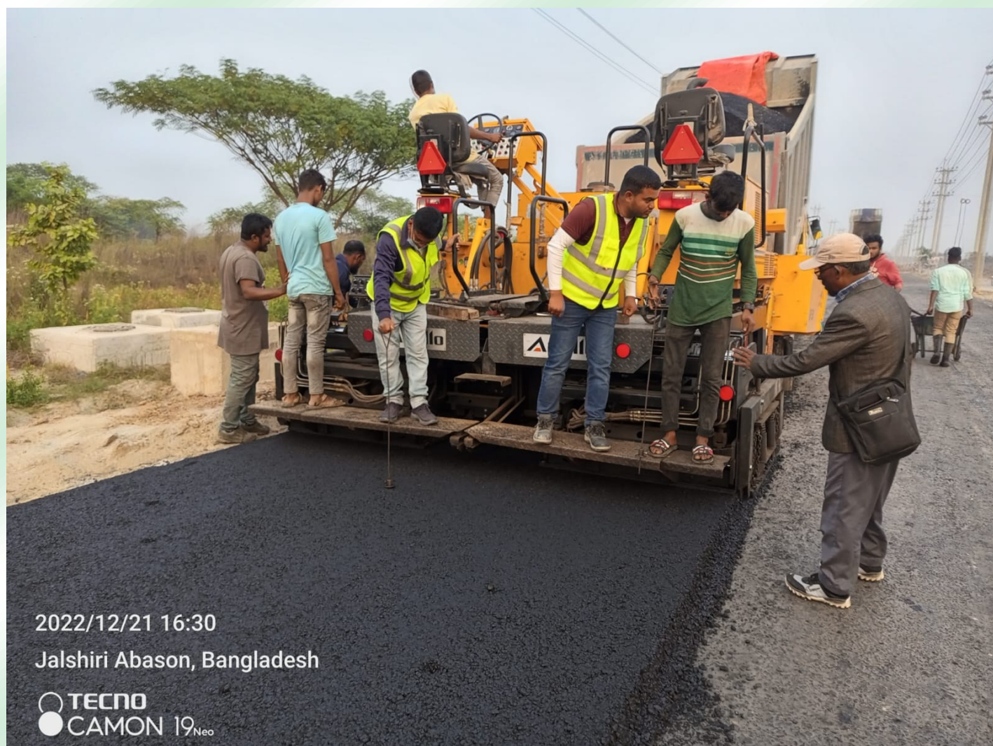
Figure: Binder Coarse at JAP Road Construction
