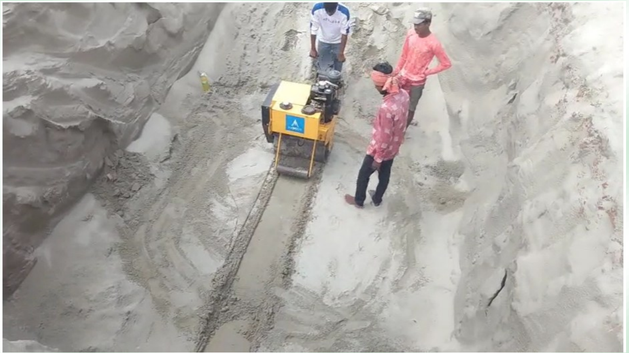
Figure: Roller Compaction at SEZL Project
