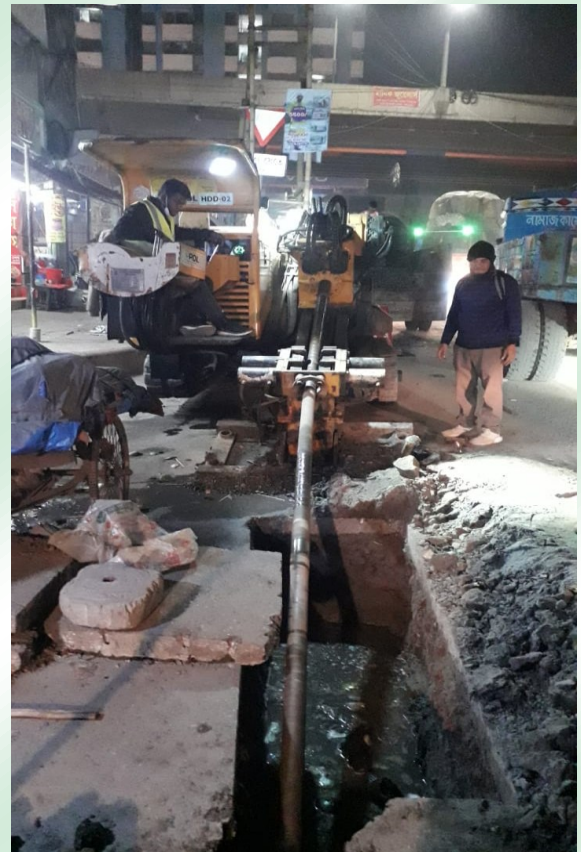
Figure: HDPE Pipe Joint at Dhaka Wasa
