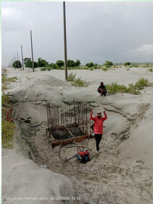
Figure: Inspection Pit Base Construction at SEZL Project
