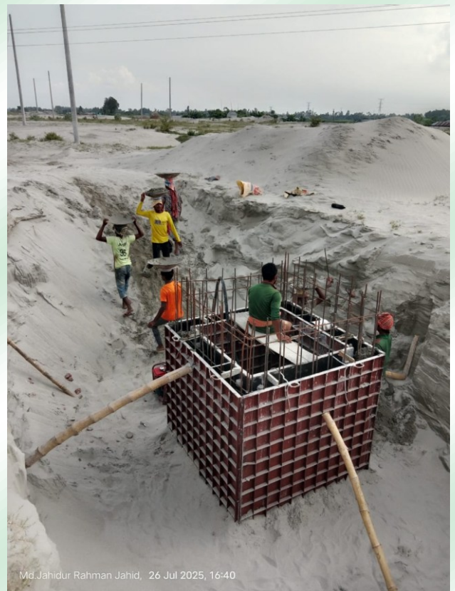
Figure: Inspection Pit wall Construction at SEZL Project
