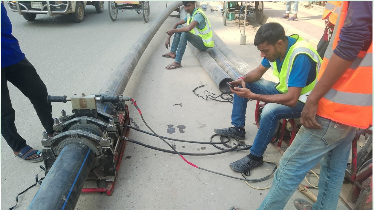
Figure: HDPE Pipe Joint at Dhaka Wasa
