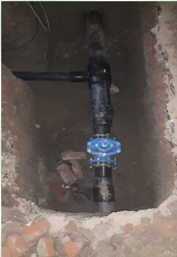
Figure: Valve Installation at Dhaka Wasa
