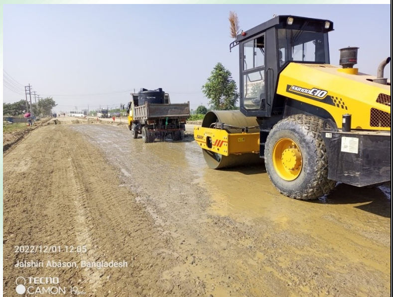
Figure: Watering at JAP Road Construction
